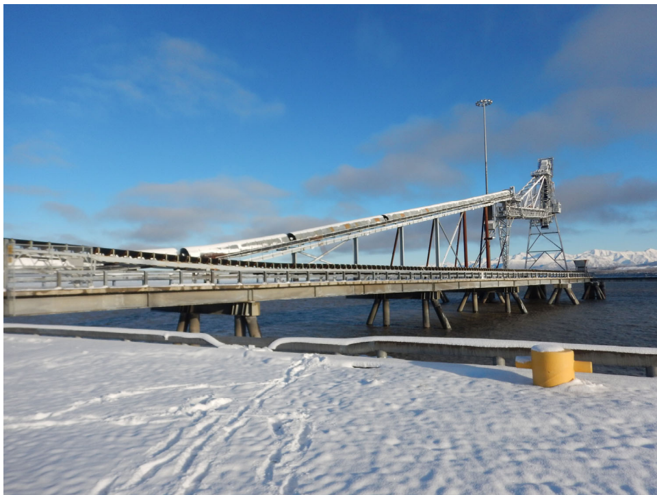
Photo 6. Port MacKenzie – Deep Draft Dock viewed from bulkhead.
