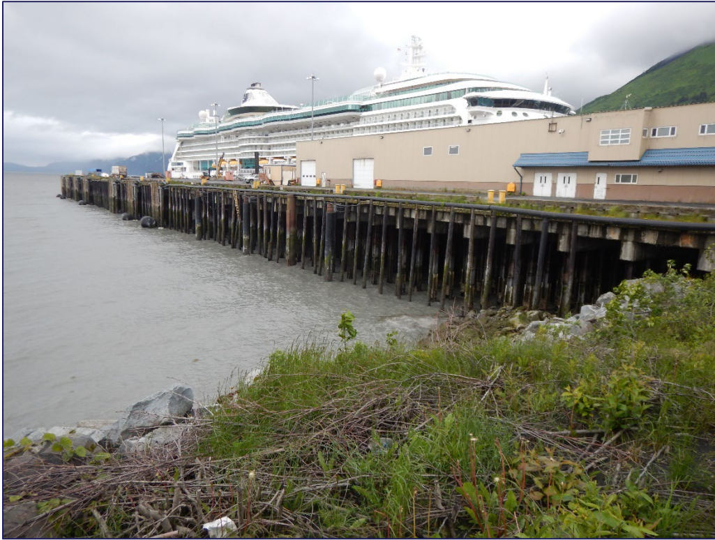
Figure 1-15. Passenger Dock Looking South
