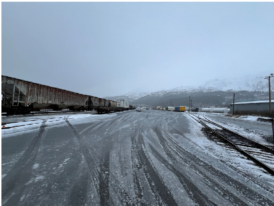
Photo 14. Whittier – Storage area between barge slip and main tracks.
