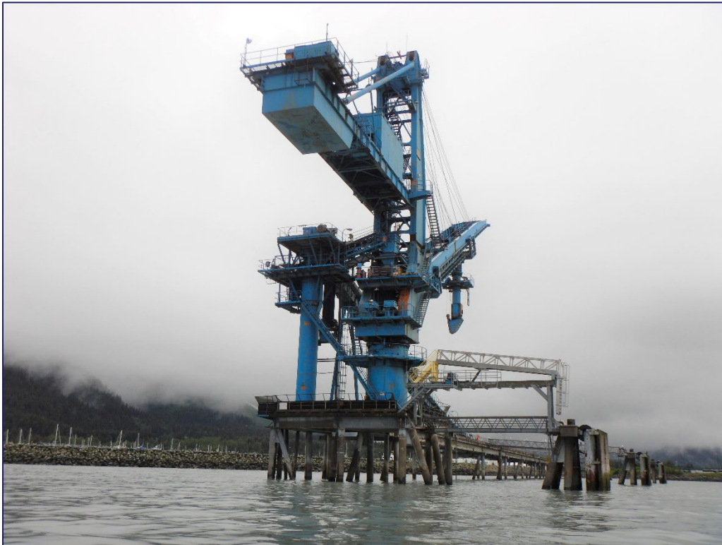
Figure 1-14. Coal Dock Looking North
