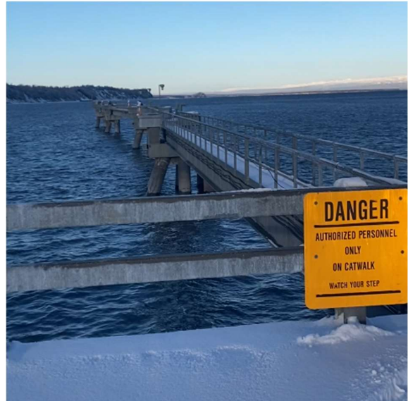
6. Northern Catwalk and Dolphins
