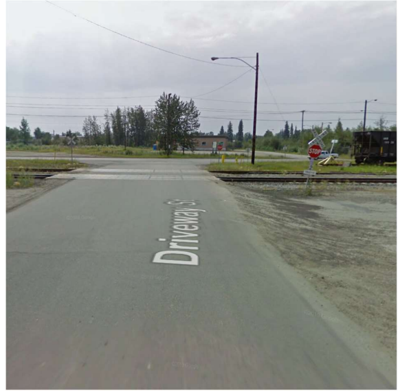
6. Rail on Driveway St, Before Phillips Field Road (taken from Google Maps due to obstruction of view due to snow)
