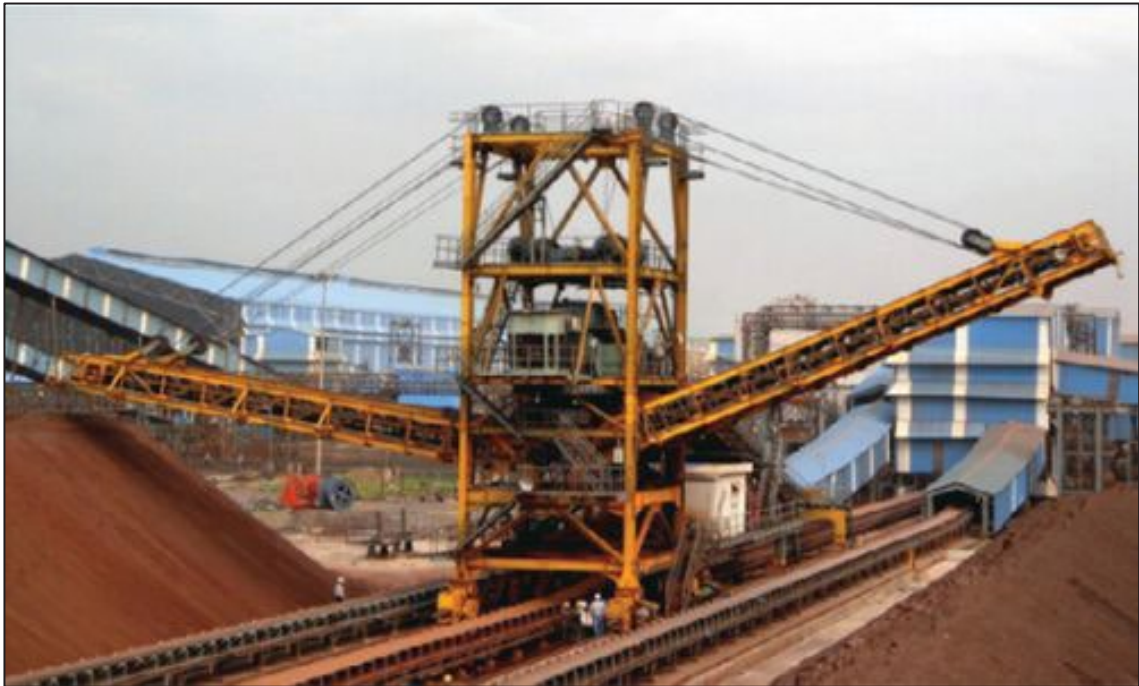
Figure 6-5: Auxiliary Twin-Boom Coal Stacker
