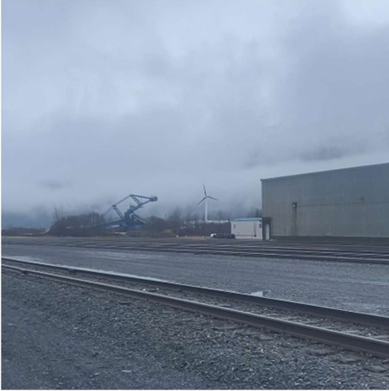
1. Rail Track to Port & Coal Stackers/Reclaimer
