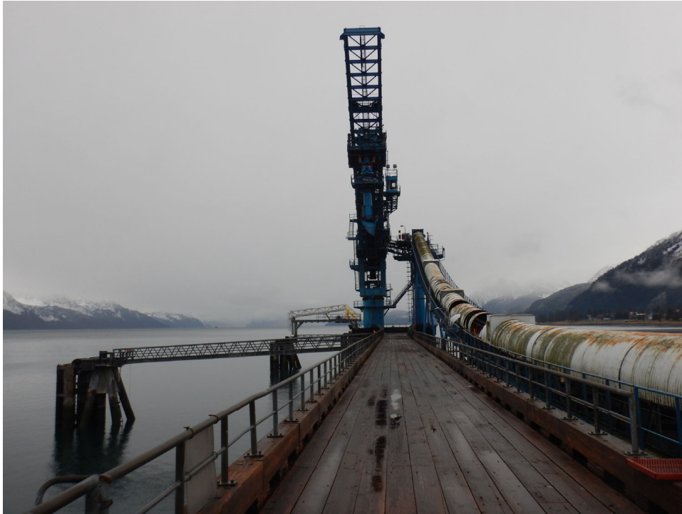
Photo 15. Seward – Coal Dock and loader arm.
