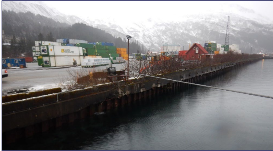
Figure 1-9. Existing Marginal Wharf (Note Only Seawall Portion Remains)
