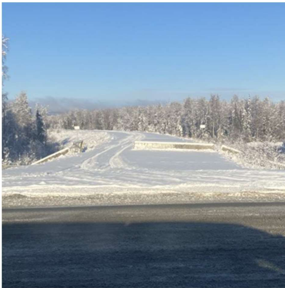
1. Partially Completed Rail Embankment Example
